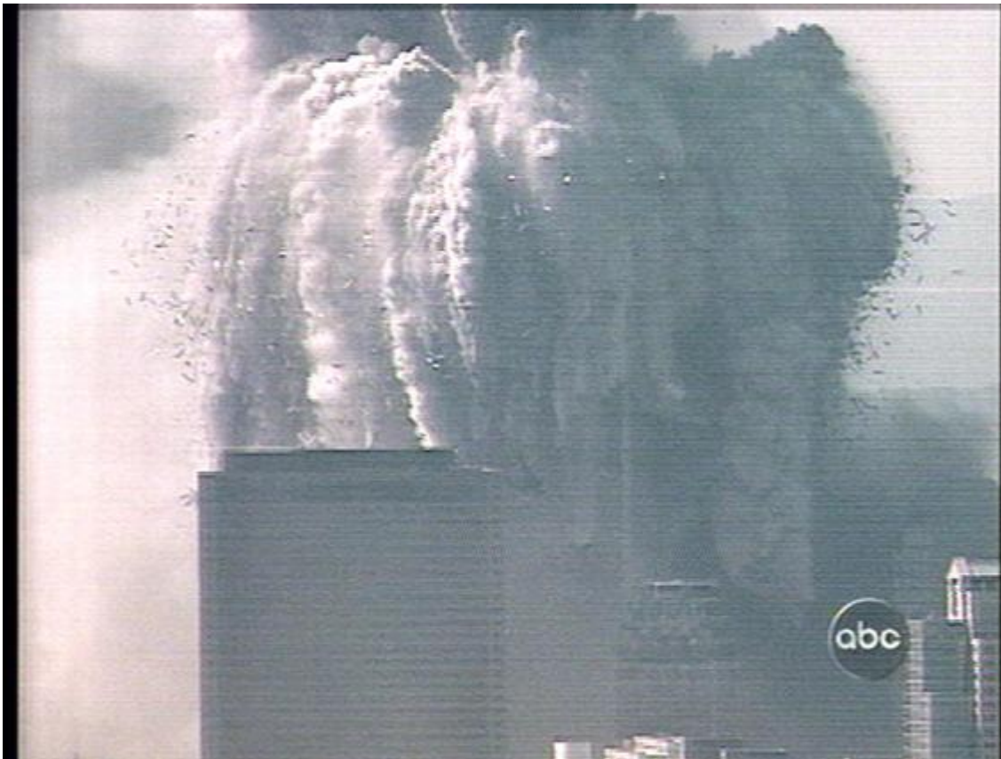
Signed by the uniform demolition mode. Lend wings to steel debris, and you get the windy towers of 9-11 as they collapse.
